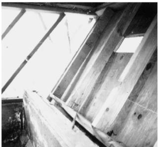
**Figure 23** - This photograph shows an interior detail of a home similar to the one above, showing substantial damage to a building with an unbraced tall wall.
