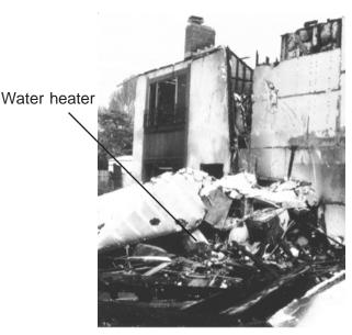
**Figure 10** - The unbraced water heater in this home fell during an earthquake; the resulting fire destroyed the home.
