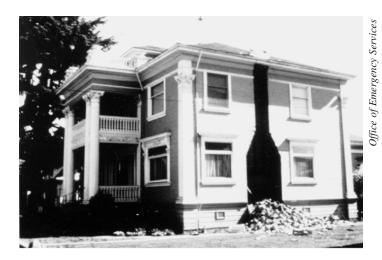
Figure 33 - This unreinforced chimney fell during a recent earthquake.
