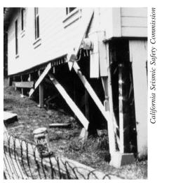
**Figure 18** - The pier-and-post foundation under this home shifted during a recent earthquake.
